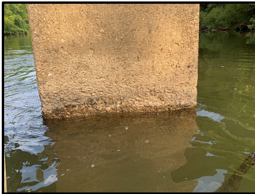
Photo 10: Scaling at Waterline (Typ.)
