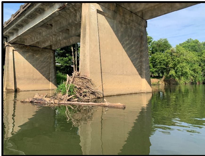
Photo 6: Pier No. 2 Looking Back At Drift Debris on Upstream Nose
